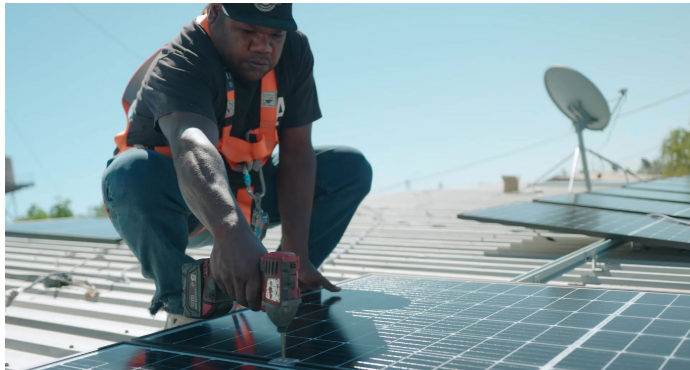
Original Power's Terry Collins installs solar panels in the remote Northern Territory community of Marlinja
