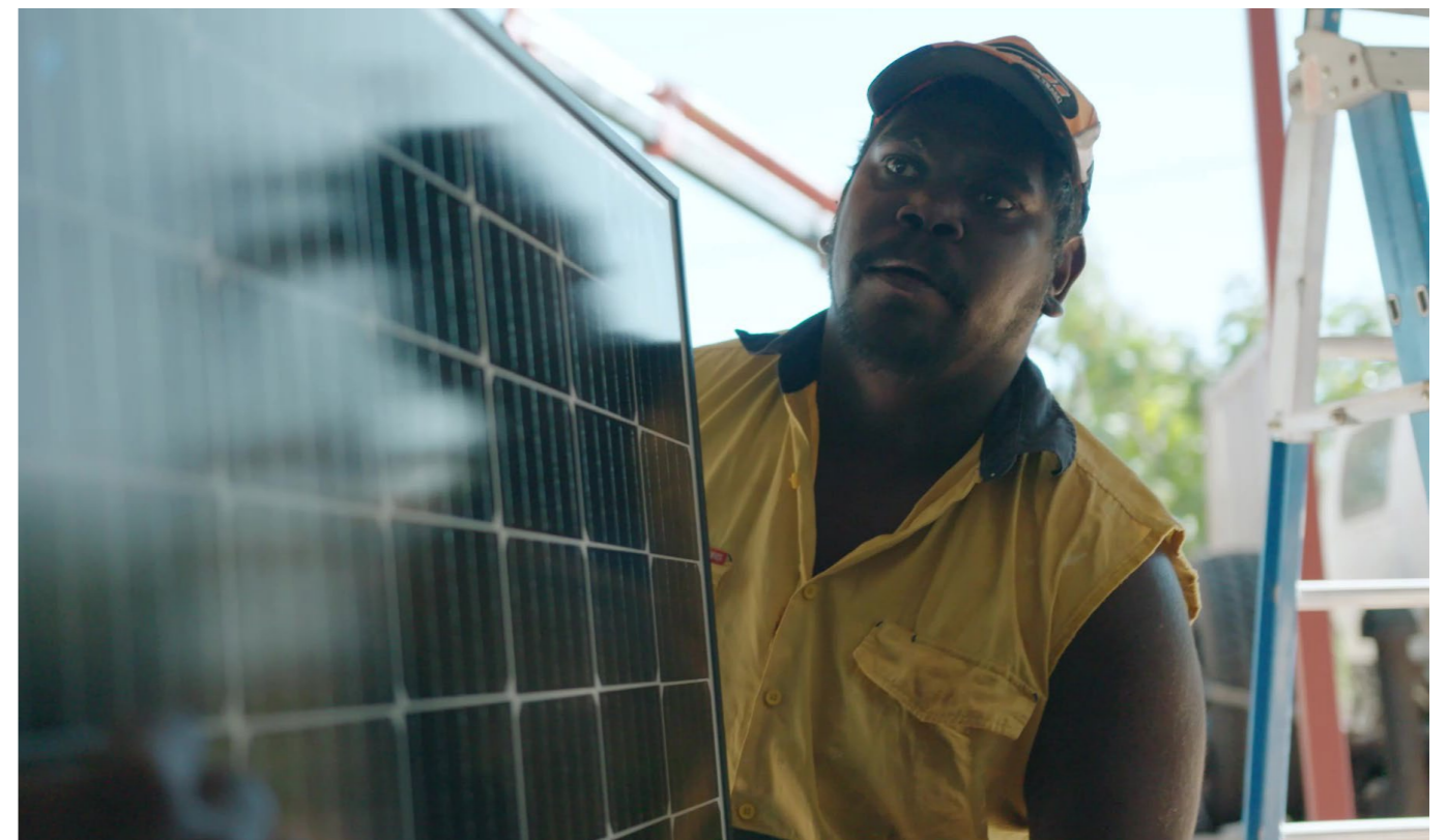
First Nations Clean Energy Network's Ethan Godfrey installing solar at Marlinja
