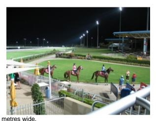
Both tracks are illuminated with the largest single floodlighting installation ever completed in Australia. The lighting provided by 900 x 2kW floodlights mounted on poles, ranging from 20 to 40m high. The lighting scheme meets the necessary brightness and uniformity required for television coverage, while providing safe and comfortable conditions for jockeys, horses and officials.
