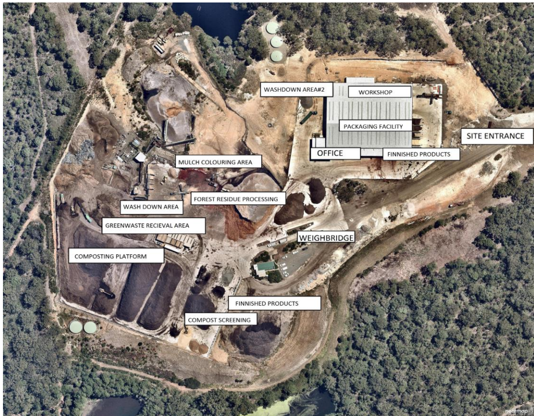
Figure 1 – 12 Pindimar Rd, Tea Gardens, NSW 2324
