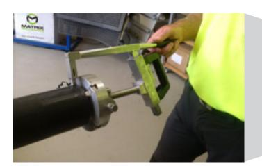
2. Scrape the outside surface of the spigot for at least half the socket length, immediately before assembly & welding. Complete and even removal of 0.2mm to 0.3mm is absolutely essential. Use a rotary scraping tool as it removes a consistent amount of material
