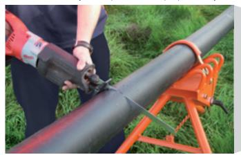
Pipe must be dry cut so that pipe ends are kept free of oil or any other contaminant. Cut must be straight to allow full insertion into EF fitting.
