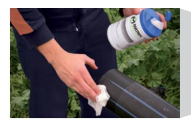
Clean the spigot and socket interior with alcohol wipes, and allow to completley dry. Ensure spigots & socket interior are dry and free of any contamination before assembly. Retain EF fittings in their original bag until ready to weld.
