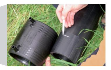
5. Be sure the joint is kept straight, still and not under any stress during weld and cool down time. Must not be artificially cooled in any way. If you have any further questions please call one of our helpful staff on 1800 634 644.
