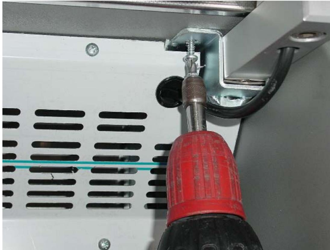
**17)** To fix the service plate, you'll have to screw by the exhibition part, the necessary points ( 2 or 3 in accordance the the cabinet width).
