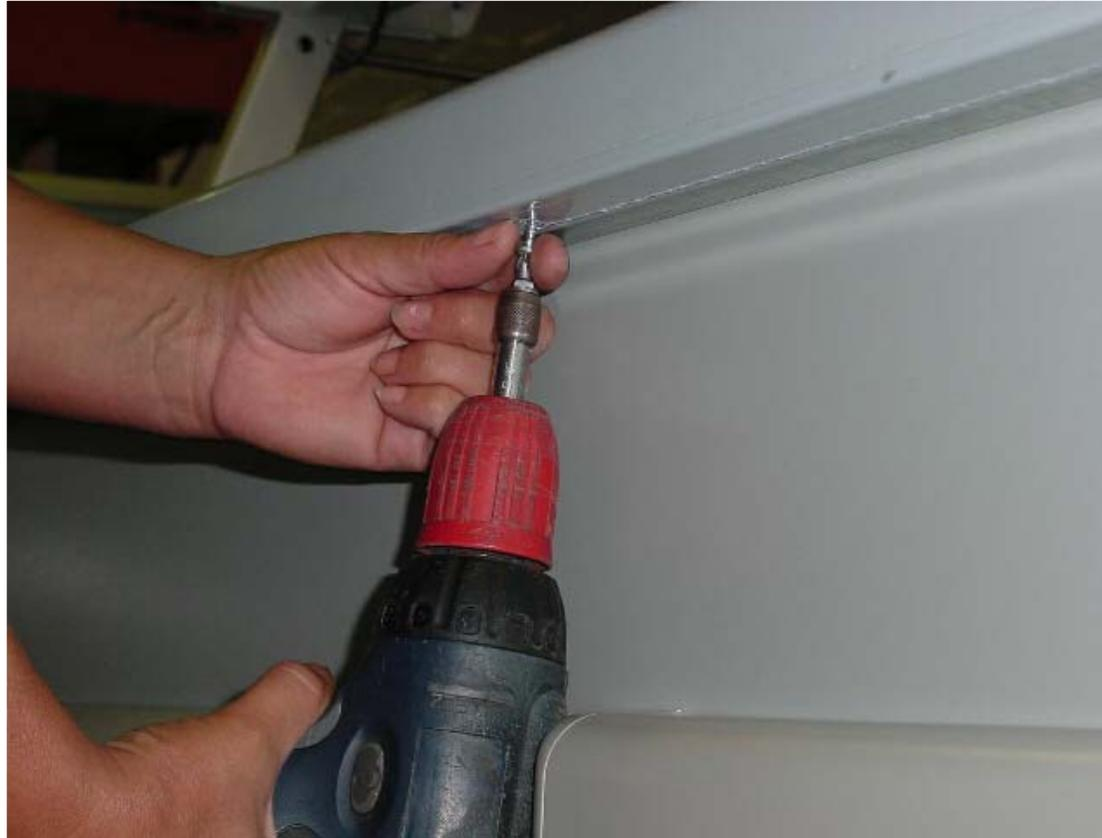
**18)** Fix the service plate on the backside of the cabinet as shown.
