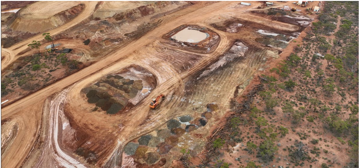
Figure 4: Lucky Strike ROM Pad at 0800 on 7 April 2026
