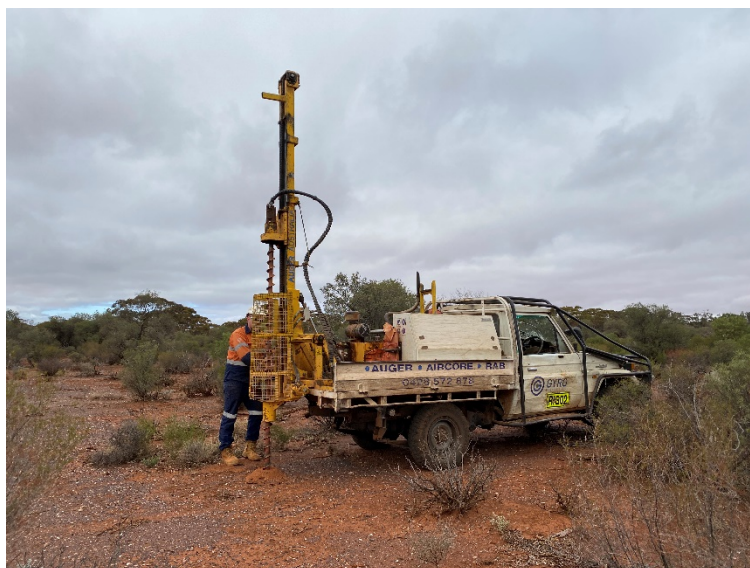
Auger drilling along the Mt Monger Trend
