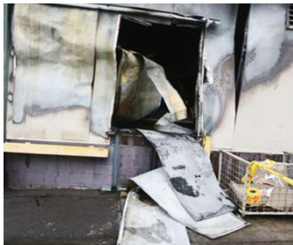
B = Fire Brigade accessed fire by cutting through exterior
