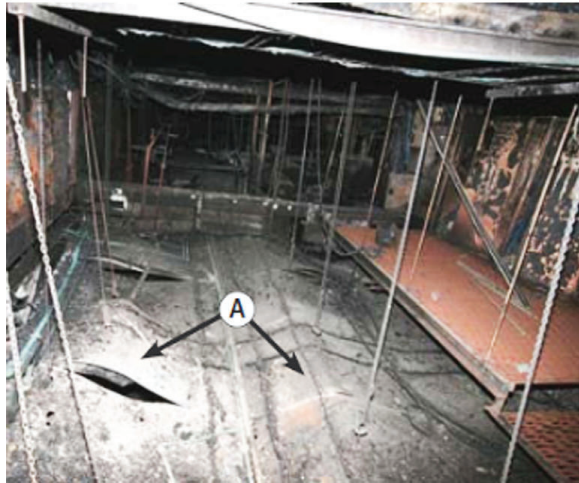
A = EPS panelling and 3m roof void Fire undetectable below roof void
