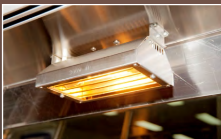
Quartz infra-red overhead heat lamps
